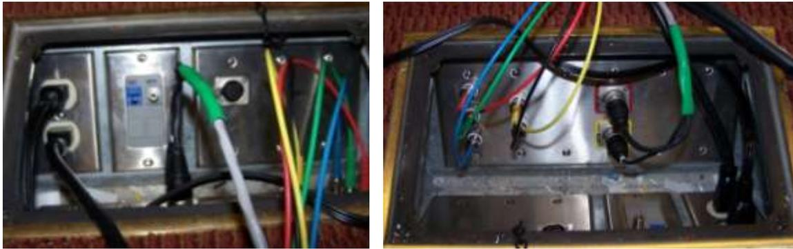
1. Attach the main power cord into an outlet in the floor panel.
